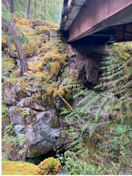
Left Bank Abutment when facing downstream
