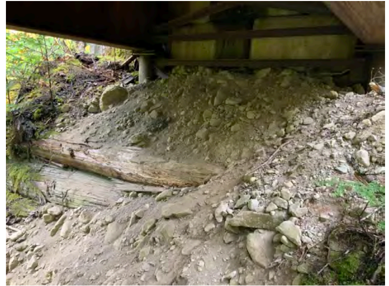
Right Bank Abutment when facing downstream
