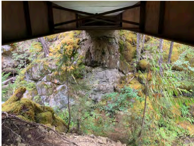
Left Bank Abutment when facing downstream
